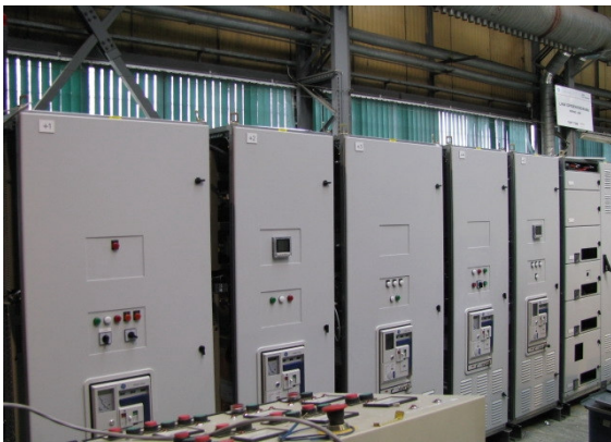
FACE A (TGBT - Phase de construction)
